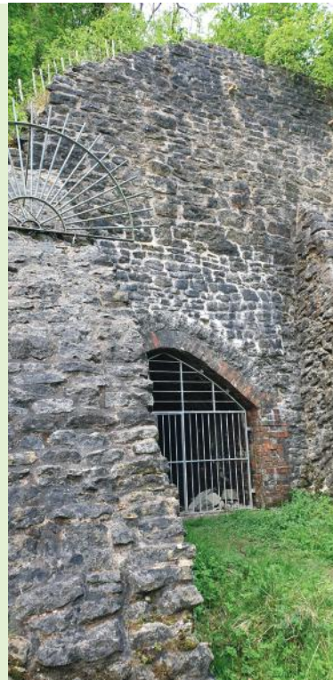
The lime kilns were originally built during the mid 1800s and operated until the 1870s, after which they fell into disrepair. A date of '1928' is inscribed above the kiln arch, indicating a date when this kiln was repaired and put into production again in the 1930s.
